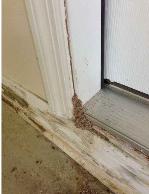
Fig. 1. Subterranean termite tube at PMU House back door. Mud tubes are evidence of subterranean termite infestation.
