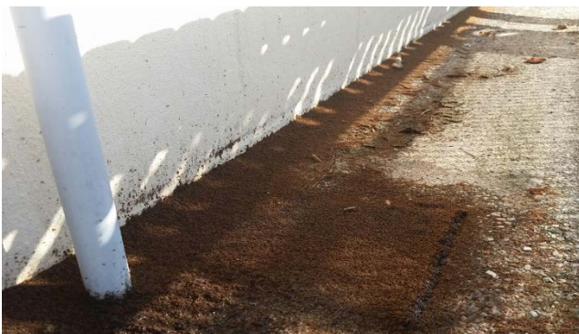
Fig 2. Dead tawny crazy ant ( Nylanderia fulva ) workers along the foundation of a treated structure. Photo: Michael Bentley, University of Florida.
