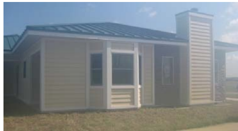
Fig. 1. Side of house with two different coverings, bay window and chimney.
